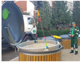
Figure 8: Connecting the hook to lifting bands
