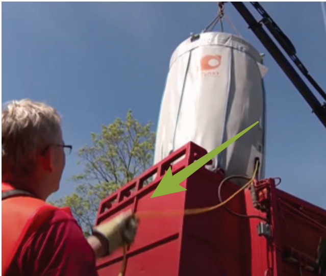
Figure 10: Emptying the bag by pulling the rope
